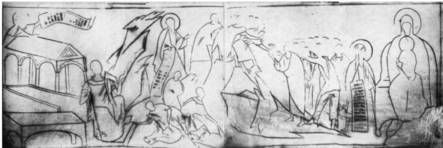
Fig. 4.2. 'Wisdom has built her house', fresco in the narthex, Dormition church in the Volotovo Field near Novgorod, 1380s, destroyed during the Second World War. Drawing by F. M. Fomin, 1894–1895.
